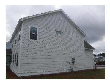
Have builder install the trim around the left side top window and replace any damaged siding to prevent water/damage to occur as soon as possible
