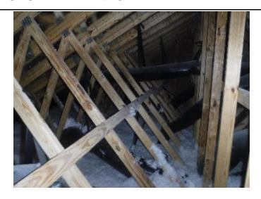
13.5  $\pm$ -inches of blown fiberglass insulation is present in attic and is rated at R-30 $\pm$ -. This meets current standards
