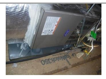
Have builder secure the a/c duct that was against the metal flue for safety and also trim the roof tar paper at the roof where pipe is also touching. Minimum of 1" clearance for safety
